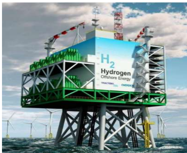
Figure 6 Bottom fixed foundation example a centralized electrolyzer
