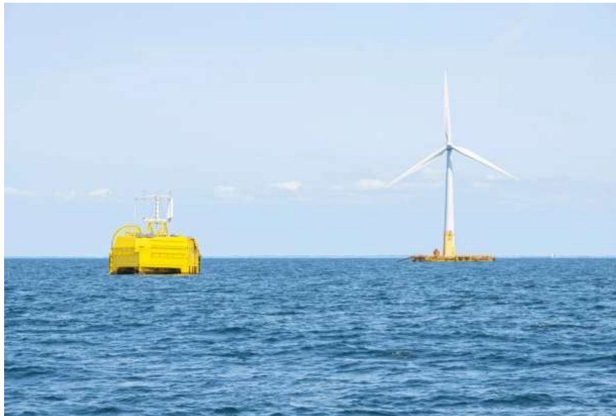
Figure 12 SEM-REV test site: (2 MW) FOWT connected with H2 electrolyzer floating substation
