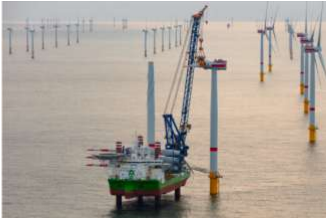
Figure 0-5 Jack-Up Vessel in operation. Source: (28).
